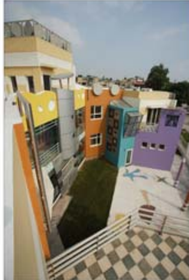
COURTYARD VIEW FROM FIRST FLOOR
