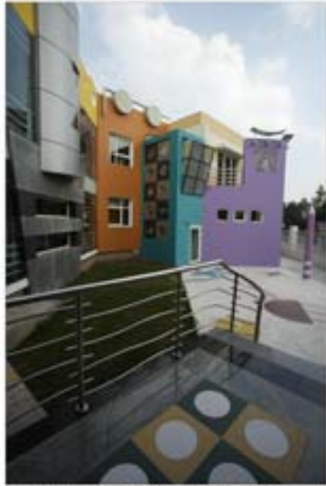
COURTYARD VIEW FROM LANDING USE OF MATERIAL CREATES TRANSITION BETWEEN DIFFERENT SPACES AS IN FRONT COURTYARD COLORFUL ABSTRACT SHAPES CREATES VISUAL DELIGHT
