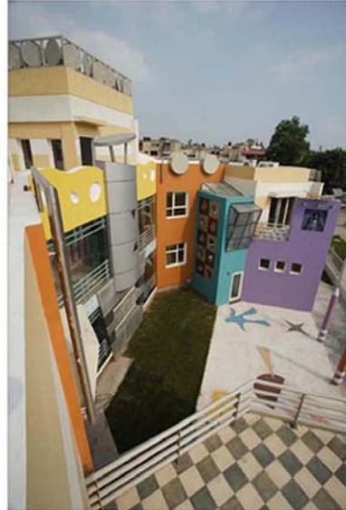
COURTYARD VIEW FROM FIRST FLOOR
